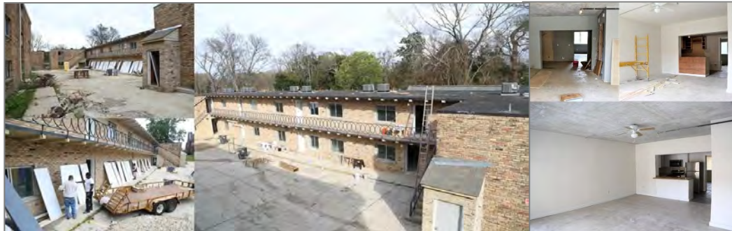
Rental units in Louisiana being repaired under Multi-Family Lease and Repair to house eligible applicants.
